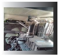
The roof and walls are insulated with rock wool and fibrous and metal protections. the whole exhaust line is coverd by insulation iackets, insulated divider.
